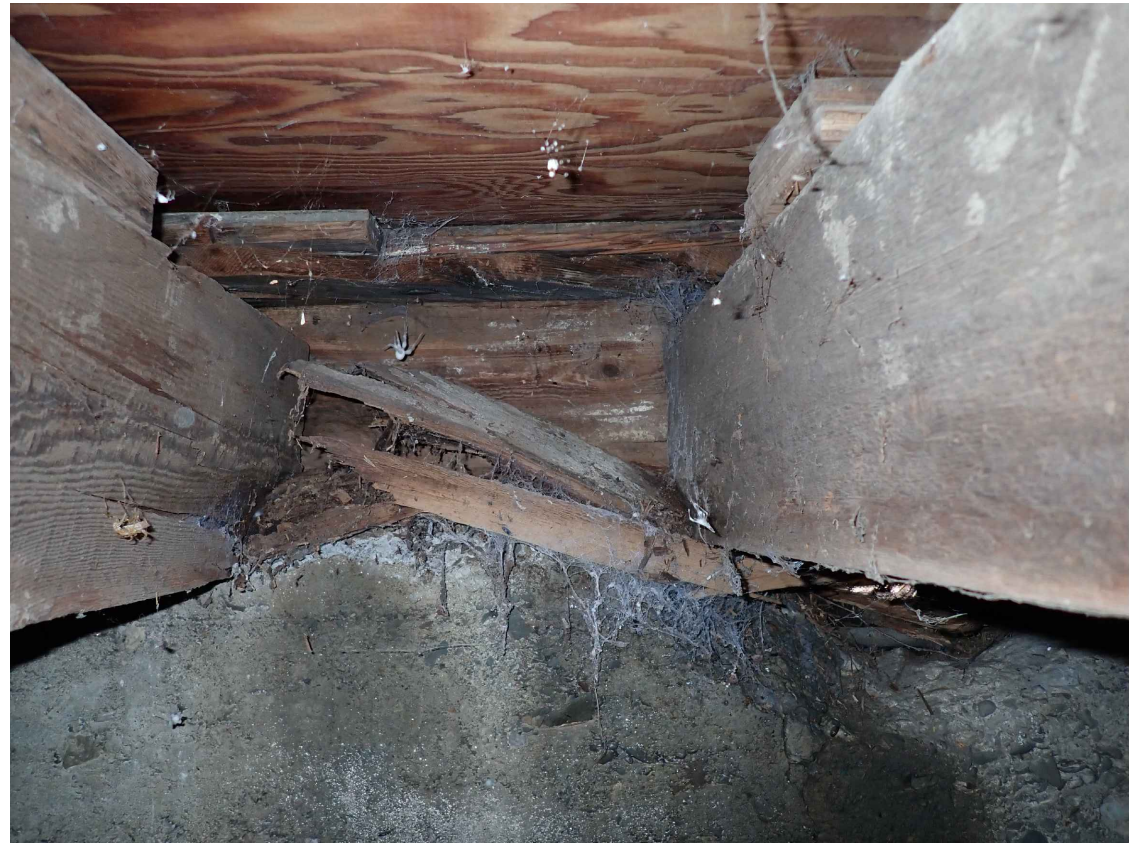
JACK UP FLOOR JOISTS AND REMOVE ROTTED SILL. PROVIDE PRESSURE TREATED 2X6 SILL APPROXIMATELY 12 FEET, FIELD VERIFY EXACT LENGTH. PROVIDE NEW ANCHORS TO SECURE SILL TO FOUNDATION.
