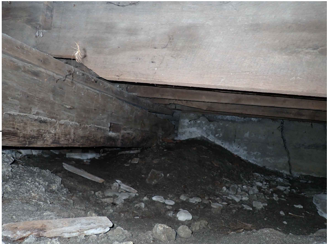
JACK UP 10x12 BEAM AND PROVIDE 16"x16" CONCRETE COLUMN TO SUPPORT. (TYPICAL IN 6 LOCATIONS, ONE ON EITHER SIDE OF THE 3 BEAMS)
